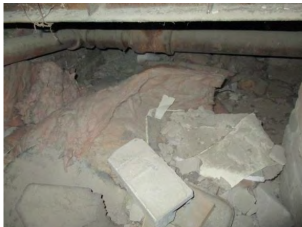
A view looking along the side of the boiler. Fragments of pipe insulation (Chrysotile 60%) and debris were observed on the floor.
