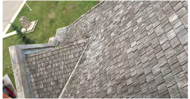
WOOD SHINGLES ON HIPPED ROOF AND GABLE DORMER
