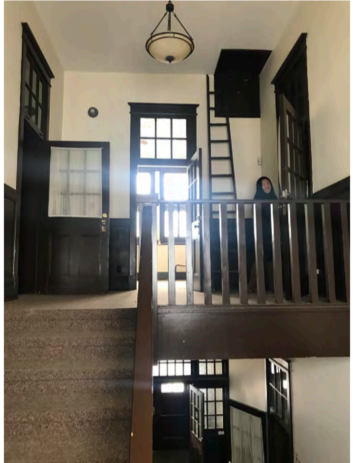
CLASSROOM DOORS AND NINE-LIGHT TRANSOMS
