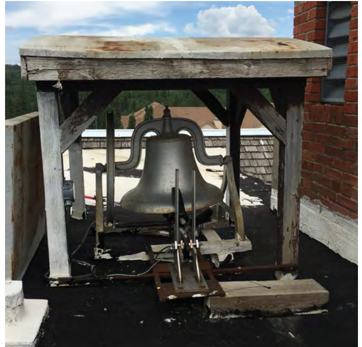
EXTERIOR BELL ON ROOF
