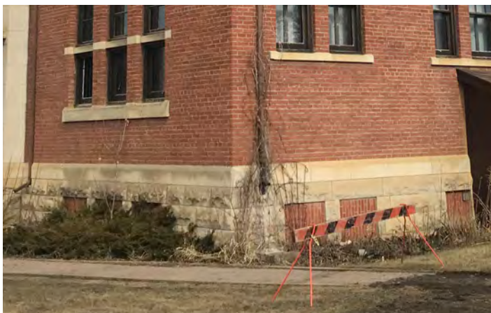
EXISTING FILLED IN BASEMENT BRICK WINDOWS
