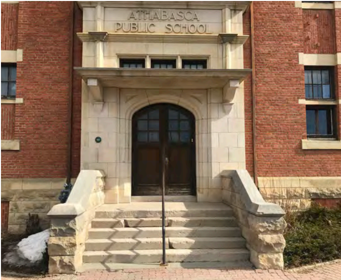
MAIN ENTRY LIMESTONE STEPS
