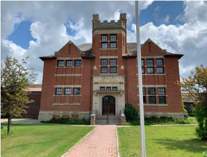
WEST FACADE, FENESTRATION PATTERN & WINDOWS ON PRIMARY ELEVATION
