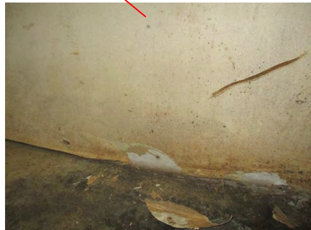
Discolouration and water staining were evident along the bottom of the drywall in the furnace room. Approximate size of affected area 110 ft 2 .
