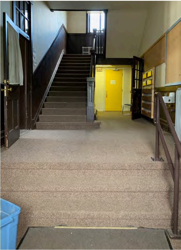
STEPS FROM FOYER TO MAIN FLOOR
