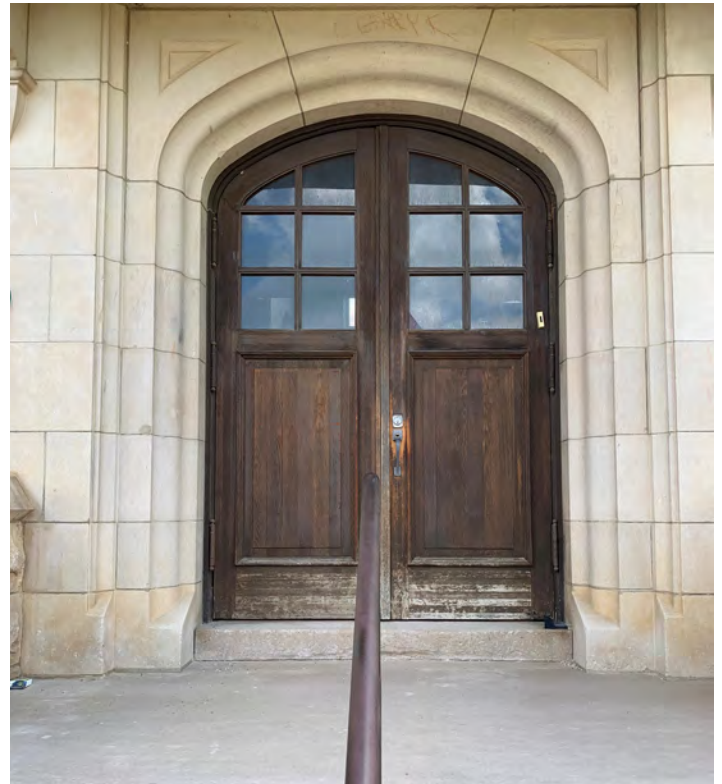
HEAVY WOODEN ARCHED ENTRY DOOR WITH SIX LIGHTS SET WITH IN A TUDOR ARCH
