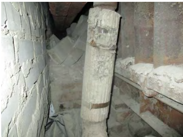
A view looking along the side of the boiler. Fragments of pipe insulation (Chrysotile 60%) and debris were observed on the floor.
