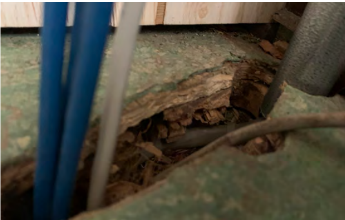
EXISTING CARPET PULLED UP
