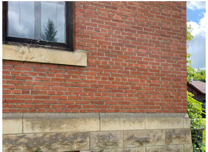
LIMESTONE BELT COURSE & ROUGH FACED STONE FOUNDATION
