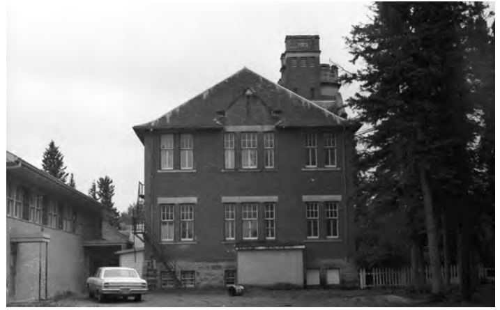
OLD BRICK SCHOOL NORTH ELEVATION WITH FIRE-ESCAPE, 1970
