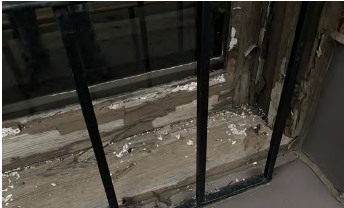
EXTERIOR WINDOW SILL
