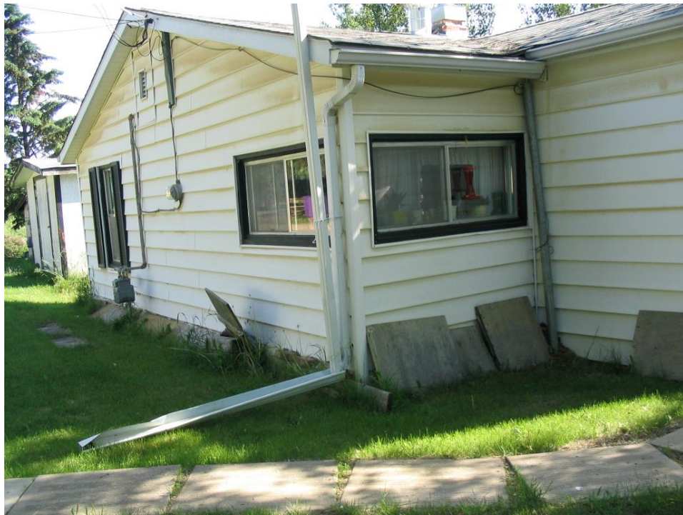
Photo 28 – Wood slabs around base of home
