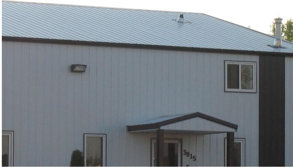
Photo 33 – Metal siding and roofing
