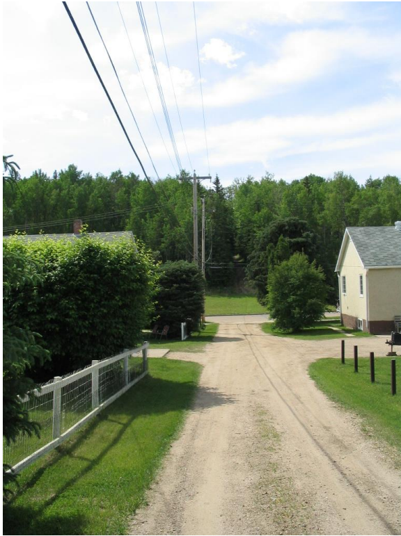
Photo 41 – Power lines overhead and clear
