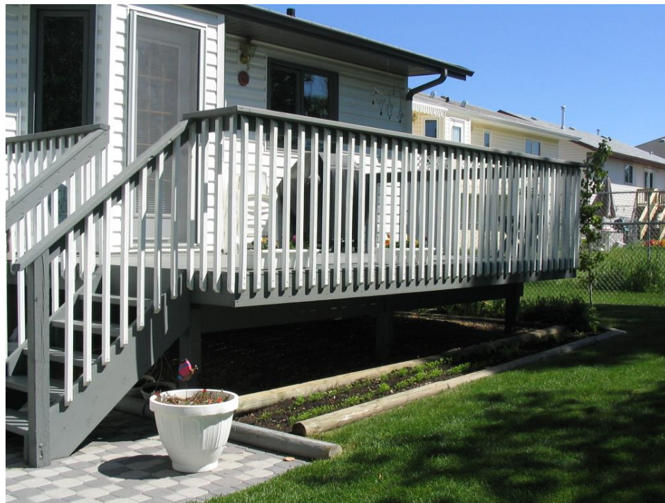
Photo 14 – Town of Athabasca, deck made of combustible material not sheathed in
