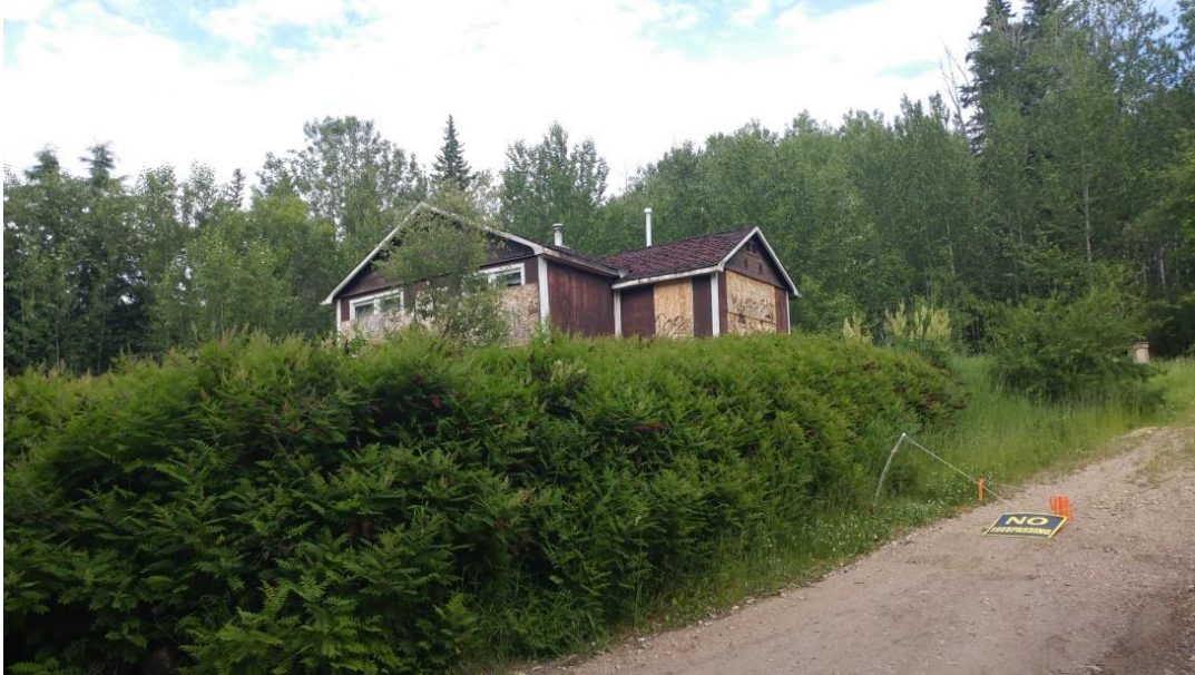
Photo10 – Town of Athabasca showing a lack of defensible space
