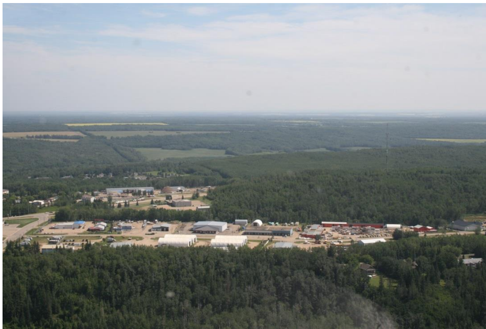
Photo 9 – Athabasca Industrial Park (north)
