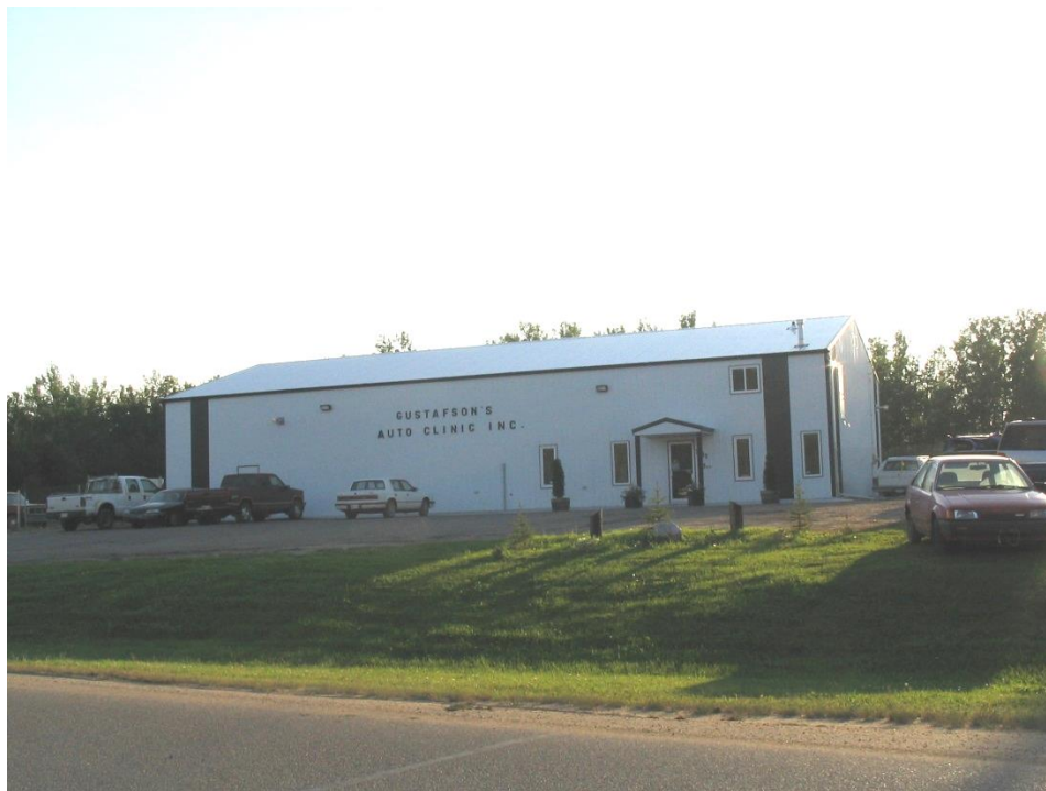
Photo 17 – Athabasca Industrial Park, metal siding and roofing, good defensible space
