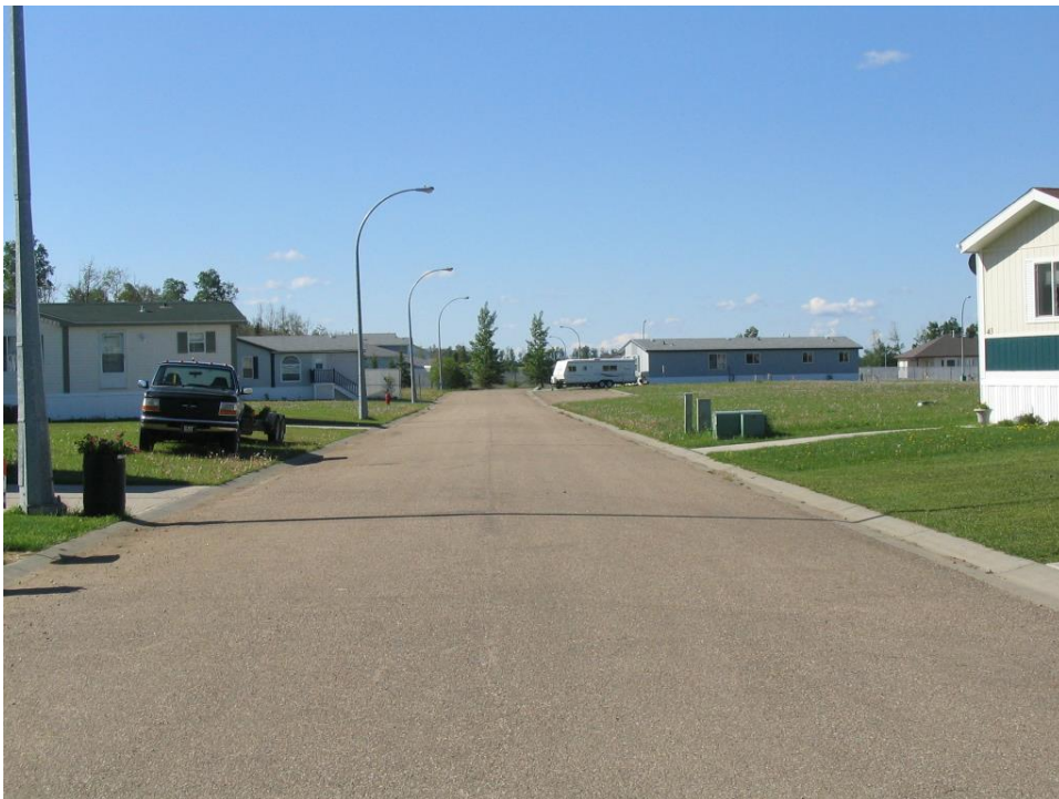
Photo 39 – Through route, wide roadway
