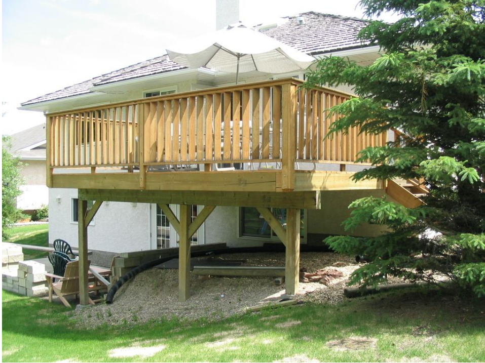
Photo 24 - Well maintained yard, structure of wood shake roofing and cement/stucco siding
